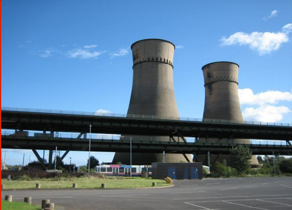
Tinsley Cooling Towers
