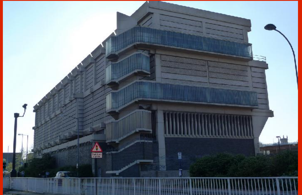
Industry: Electricity Substation, Jefferson Sheard 1968
